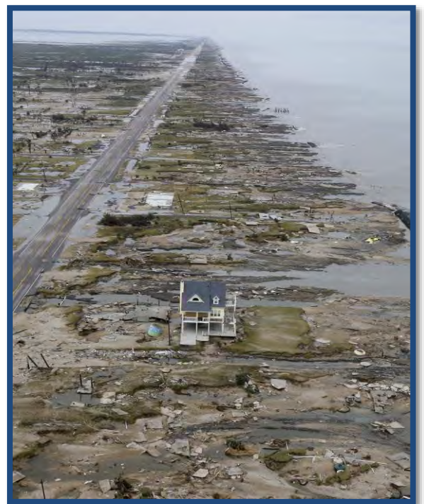
A home is left standing among debris from Hurricane Ike (2008) in Galveston County, Texas. Floodwaters from Hurricane Ike were as high as eight feet in some areas causing widespread damage across the coast of Texas. Photo Credit: David J. Phillip-Pool/Getty Images.
