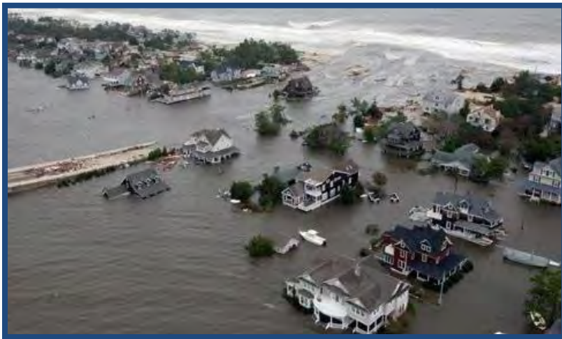
Hurricane Sandy coastal flooding in Mantoloking, NJ. Photo Credit: New Jersey National Guard/Scott Anema.
