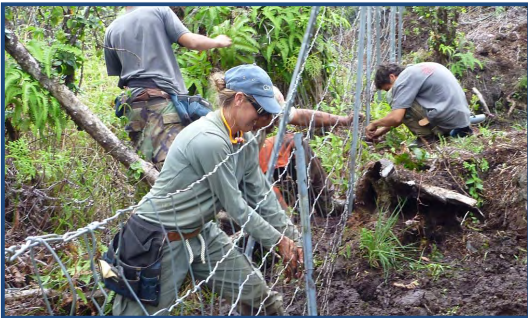
Hawaii's Watershed Partnerships construct fences in critical natural areas to protect natural resources and ecosystem services from the impacts of invasive animals. Photo Credit: Emma Yuen, Hawaii Department of Land and Natural Resources.
